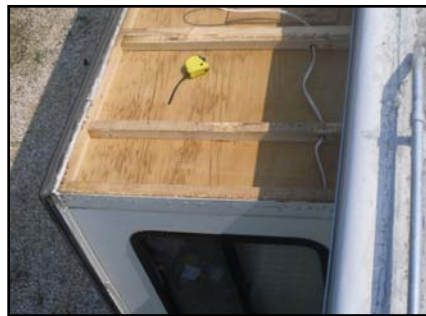
End of the summer home modification: leaky roof repairs
